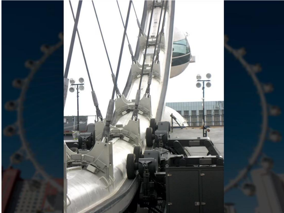
Figure 11: Hydraulic drive system for Las Vegas Observation Wheel [11]
